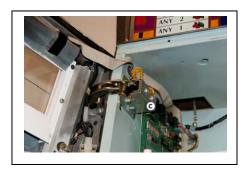
Step 3: Using a 7/16" wrench, remove D and E hex nuts on lower hinge.
